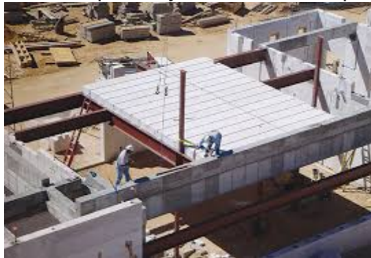
Eastland floor panel system installation process.
